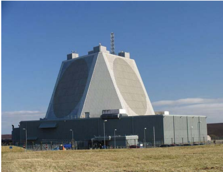
USAF PAVE-PAWS Radar ( f=0.4 GHz) 2.2° beamwidth, 2677 antennas, 22x22 m 2
